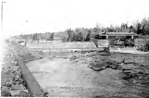
FIG. 2.—VIEW OF OLD DAM FROM BELOW.
